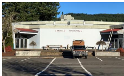
New Auditorium Roof Structures
