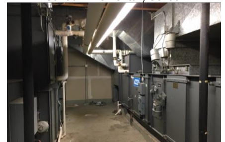
Heating/Air Flow Upgrades and Repairs Santiam Elementary School
